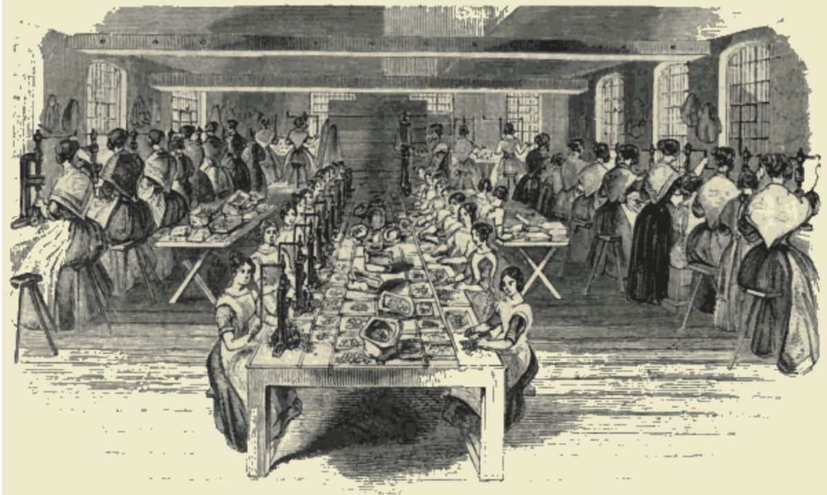
Stamping, pressing, and punching buttons.—Elliott's factory.
