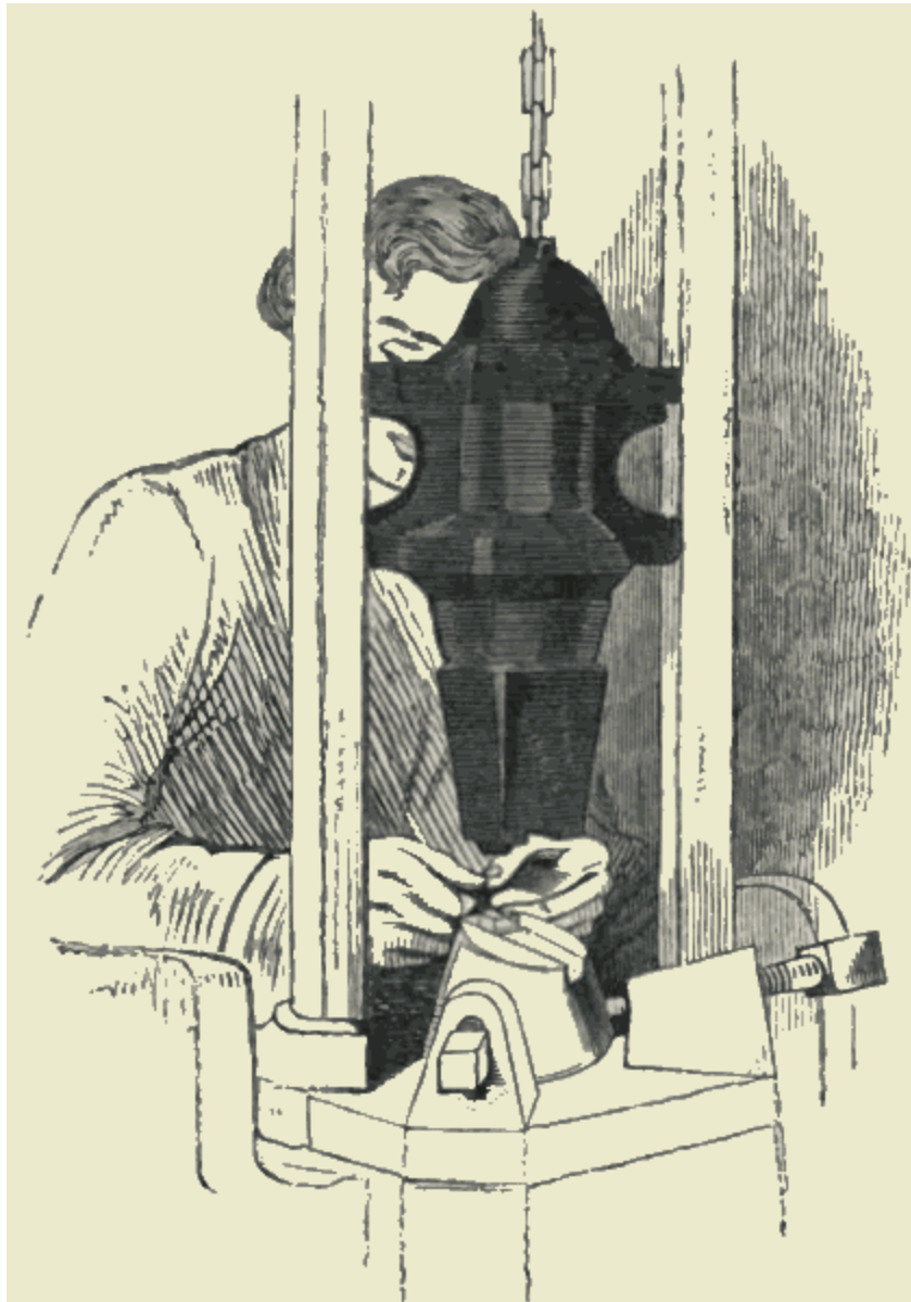
Stamping the eye of a needle.
