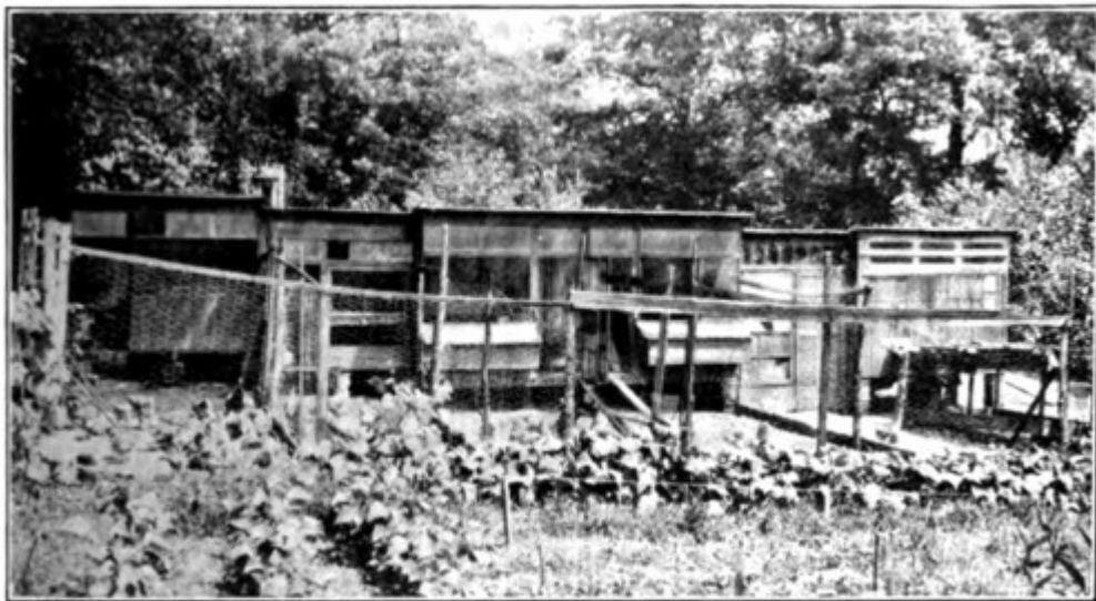
Fig. 8.—A larger poultry house suitable for a suburban lot. Notice the old lumber, sash, etc., used in the construction. The utilization of such used material, which can often be purchased for a very slight sum at auction or where buildings are being wrecked, lessens the cost of the poultry buildings very materially.
