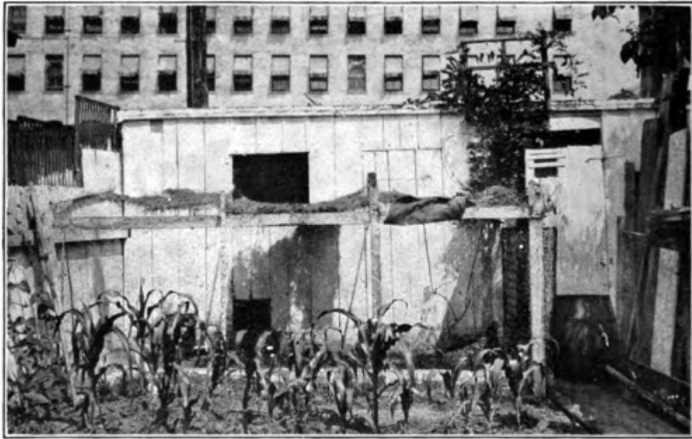
Fig. 3.—A shed in the heart of the city utilized for a poultry house. While a larger opening in the front would admit more light and make a more suitable hen house, the fowls kept here have done very well. The wire netting used for the yard was purchased very cheaply at an auction. The grass and sacks shown on the top of the run are used to furnish shade.
